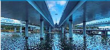
Smart Treatment for Water
